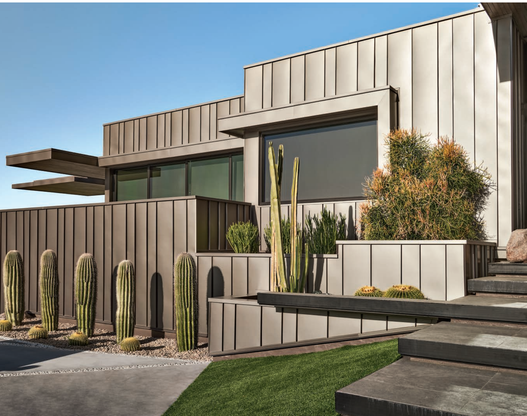
Inspired by their collection of contemporary art and design, homeowners Dimitri and Suzanne Haniotis worked with interior designer Lynne Beyer and architects Nick Tsontakis, Aaron Forbes and Jörg Berghäuser to create their sleek Paradise Valley oasis. The home's modern statement begins with exterior metal cladding installed by Charly's Roofing that becomes "a different color in the morning and at sunset," notes Suzanne. "It can range from brown to green, to almost a warm gold tone."
